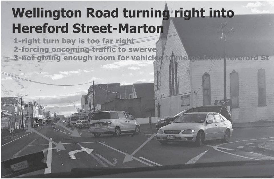
Concerned group's photo. A new cycle lane was added to the north bound side of this busy Wellington Rd intersection and pushed the centre turning lane across, to cause a dogs leg for oncoming traffic and a sharp angle turn out of Hereford St.
