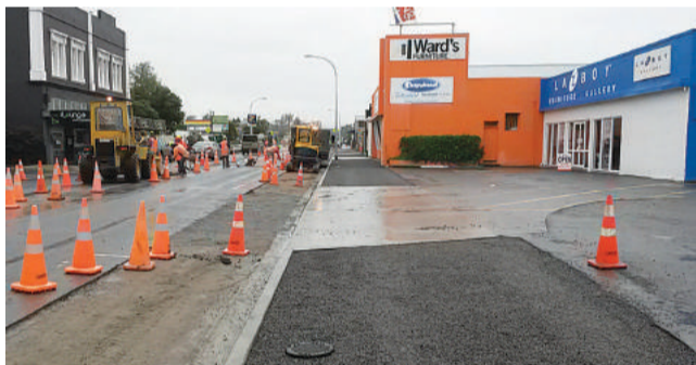
▲ Preparation of the road ready for final the hot-mix seal
