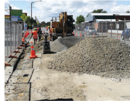
▲ Large amounts of raw materials were required for the project
