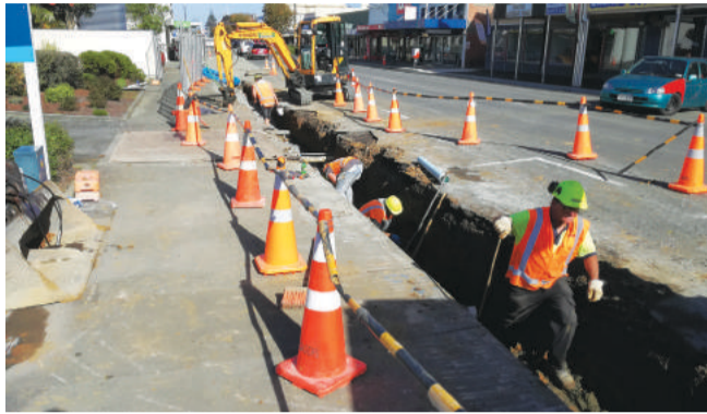
▲ A time-consuming aspect of the project was work on the water-mains
