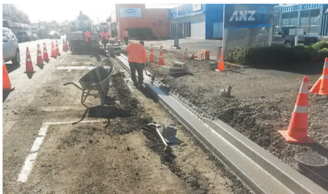
▲ Workmen laying kerb with drop crossings
