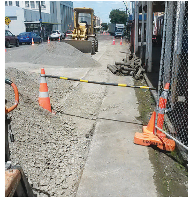
▲ The second stage of work on watermains
