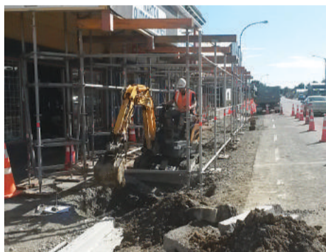
◀ Excavating beneath verandahs proved difficult at times
