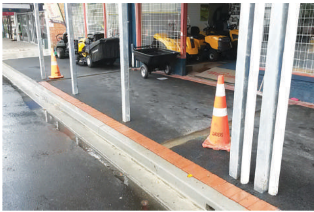
◀ The footpath outside Marton Outdoor Power once completed
